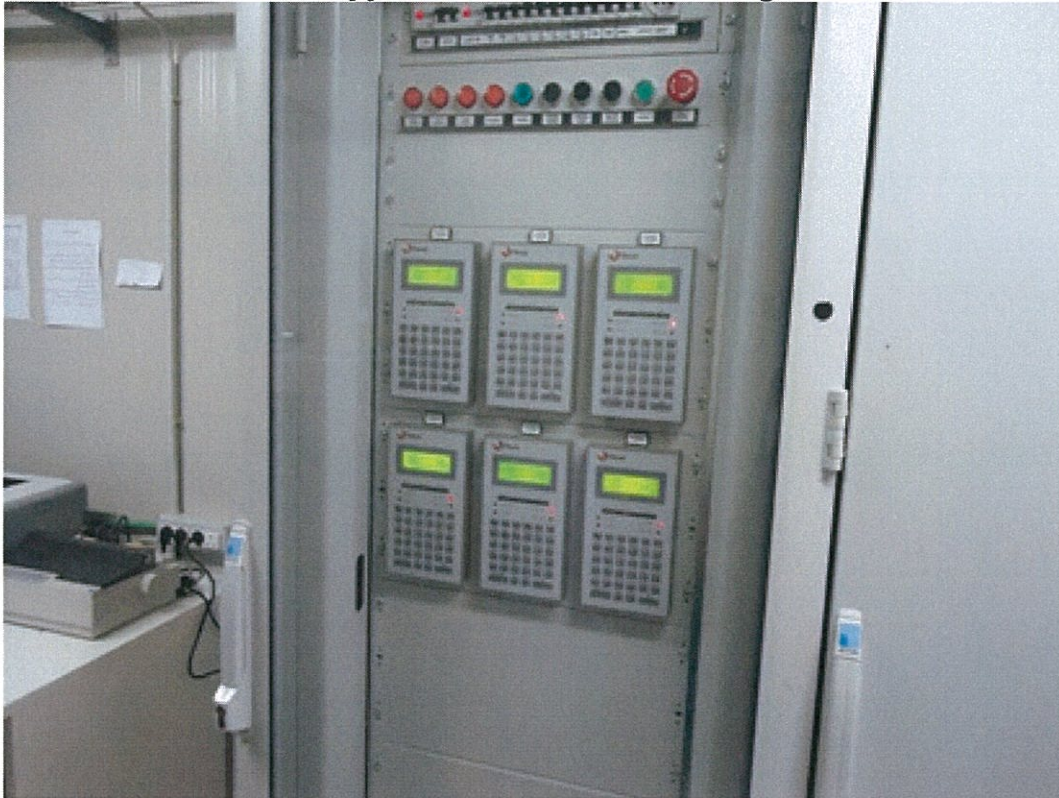
Metering Station Stream Computers
